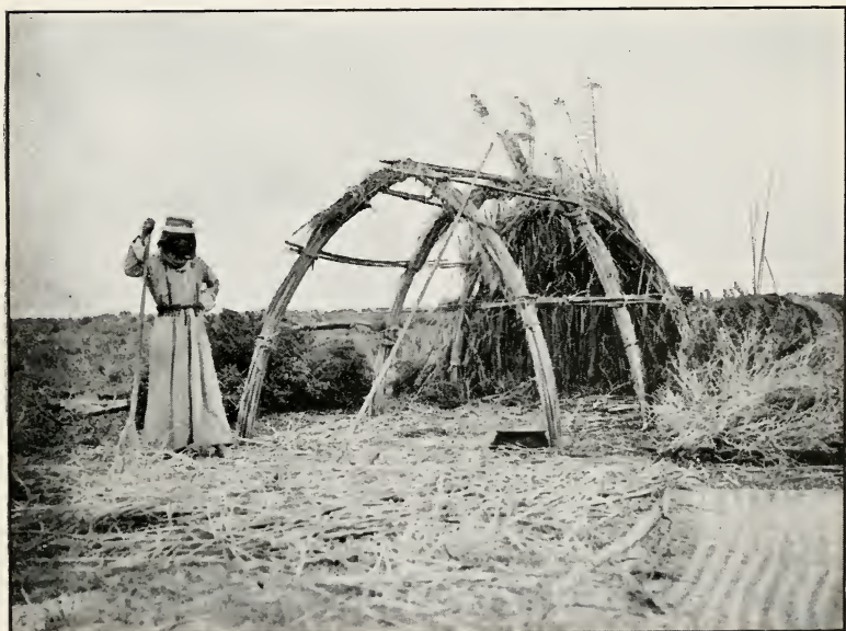
House-building in Arabistan.
